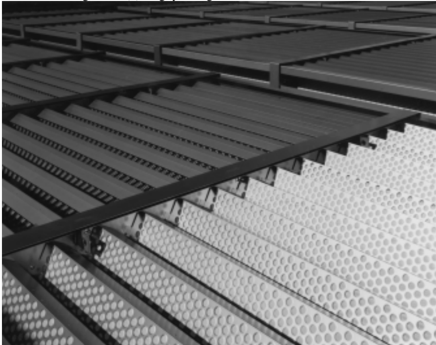
Figure 21 Detail of louver blade
