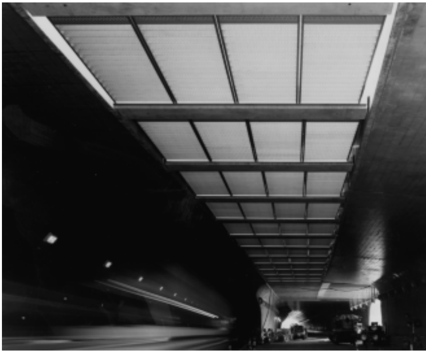
Figure 22 Louver seen from the roadway space
