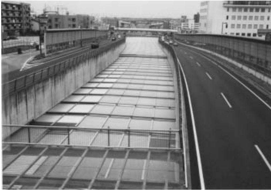
Figure 20 (b) Nagoya Ring Road after louver installation
