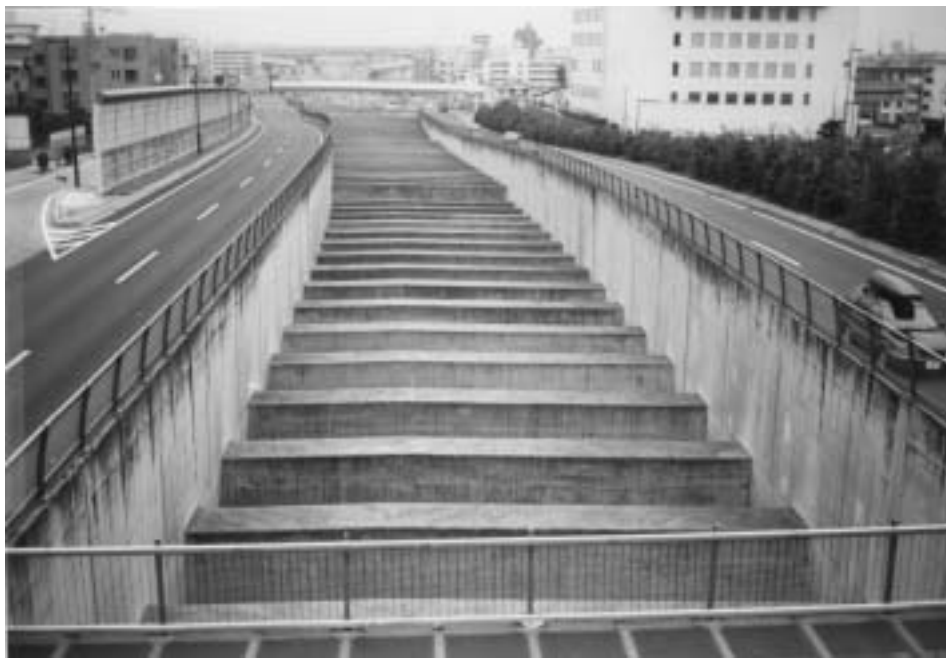
Figure 20 (a) Nagoya Ring Road before louver installation
