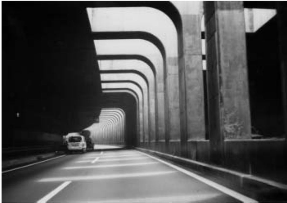
Figure 19 Visual environment in roadway space of Nagoya Ring Road before louver installation
