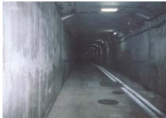
Figure 16: Service tunnel below carriage way possibility to operate small emergency vehicle)
