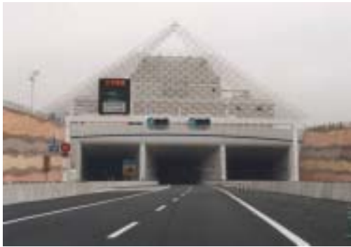
Figure 4: Ukishima Ventilation tower and entrance (west exit)
