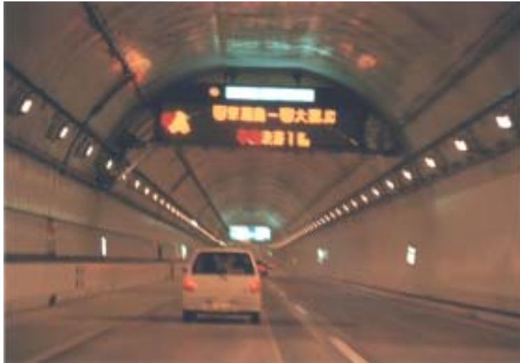
Figure 10: Whole view of the carriageway
