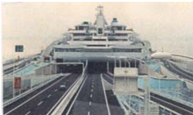
Figure 6: Kisarazu Portal on man-made island (Umi-Hotaru)
