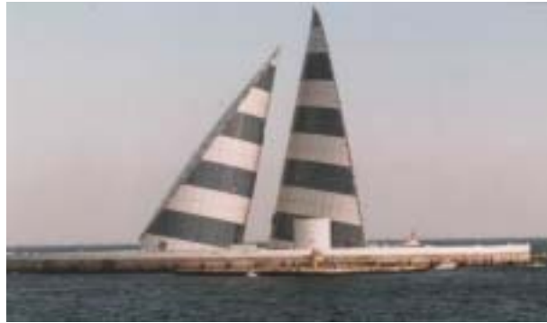
Figure 5: Ventilation tower Kawasaki Man-Made Island (Kaze no Tou)
