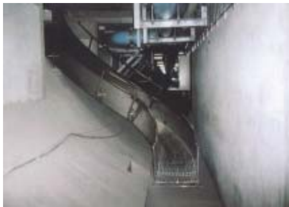
Figure 15: Slide connecting the carriage way and the evacuation space
